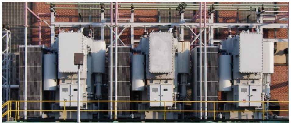
*After: Trantech cooling system with seven fans per radiator bank*
